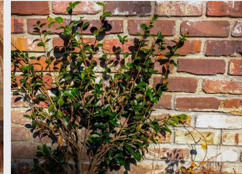
Locally produced Brick giving out an Institutional Vibe.
