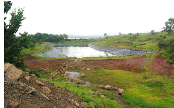
View D : Taking advantage of the existing lakes for enhanced internal views
